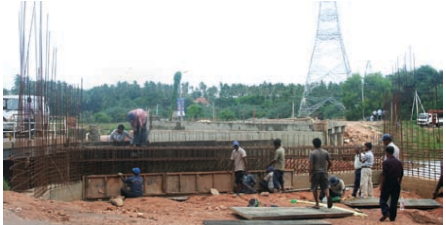
Construction of Kovinna Bridge
